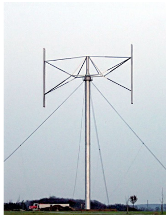
Fig. No. 06: Giromill type wind turbine [21]
