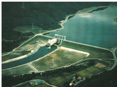
Photo 1: Tadami Power plant – a low head project in Japan
