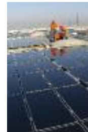
Installing thin film modules.
