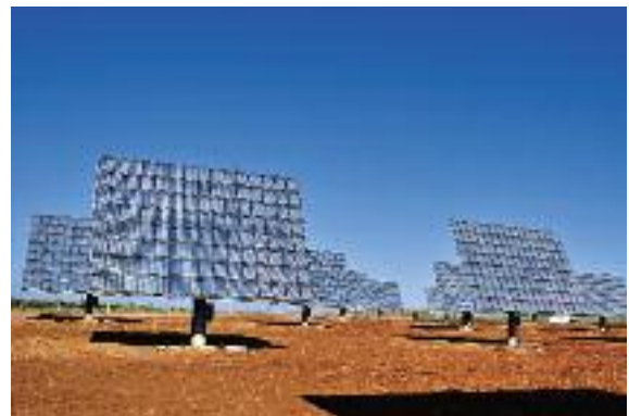
Concentrator Photovoltaics installed on trackers to follow the sun.
