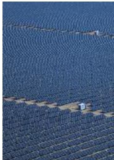
Large ground-mounted PV system in Spain.
