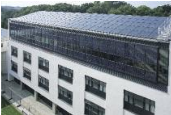
grid-connected BIPV system on the roof and façade of a commercial building.
