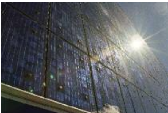
Polycrystalline silicon system integrated on a façade, St. Moritz, Switzerland.
