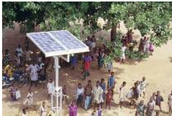
Rural electrification system in an African village.
