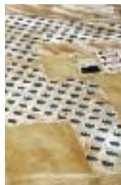
Large ground-mounted PV system in Spain.
