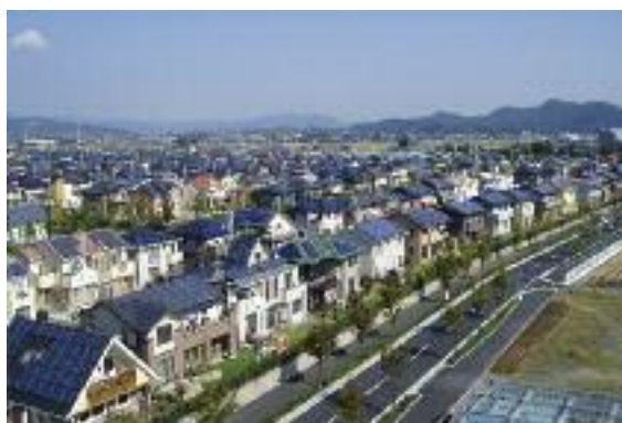
In Ohta, Japan, an interesting experiment has been conducted. The entire town has been equipped with BIPV systems to test the feasibility of a large-scale implementation.
