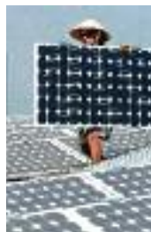
Worker installing PV on roof.
