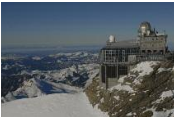
Off-grid industrial application.
