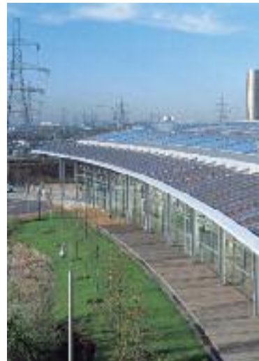
PV system integrated on a roof.
