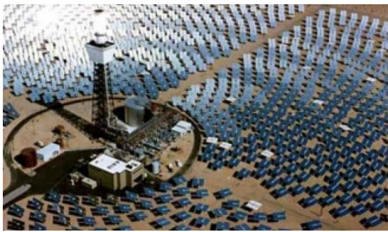
Solar Thermal: Which Technology Is Best?
