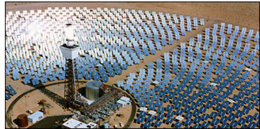
The Solar Two solar-thermal power project near Daggett, California. Every mirror in the field of heliostats reflects sunlight continuously onto the receiver on the tower.
