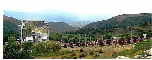
The solar furnace at Odeillo in the Pyrenees-Orientales in France can reach temperatures up to 3,500 °C (6,330 °F)
