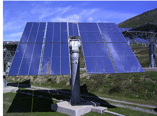
A heliostat at the THÉMIS experimental station in France. The mirror rotates on an altazimuth mount.
