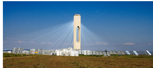
The 11MW PS10 near Seville in Spain. When this picture was taken, dust in the air made the converging light visible.
