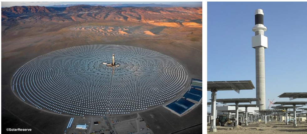
Fig. 7. Crescent Dunes Solar Energy Project in Tonopah, Nevada. (Sources: Left: SolarReserve. Right: C.K. Ho, Sandia National Laboratories).
