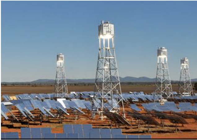
Fig. 9. Solid-based (graphite) central-receiver system at Lake Cargelligo, NSW, Australia. Source: www.graphiteenergy.com .
