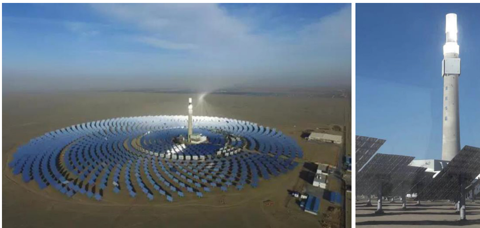
Fig. 8. SunCan Dunhuang 10 MW molten-salt central receiver plant in China with 15 h of storage. Source: CSP Focus.
