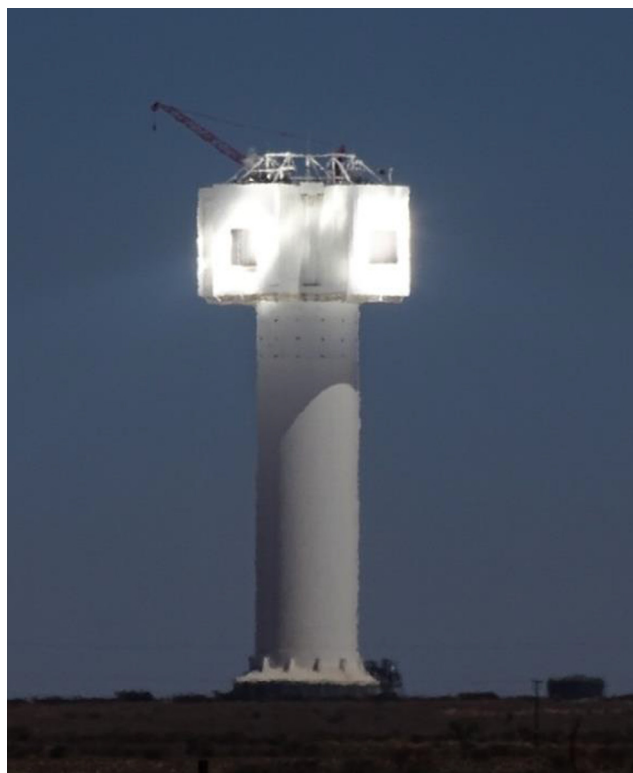
Fig. 5. Khi Solar One direct-steam central receiver system in South Africa. Source: Wikipedia Commons.
