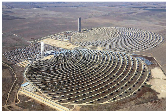
Fig. 3. PS10 (left) and PS20 (right) near Seville, Spain – the world's first commercial central receiver (power tower) plants. Source: Wikipedia Commons.
