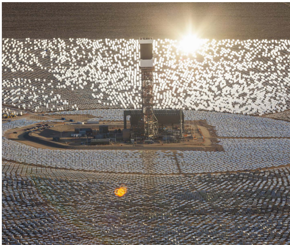
Aerial view of one of the Ivanpah power towers in Ivanpah Dry Lake, California. Photo Credit: BrightSource Energy
