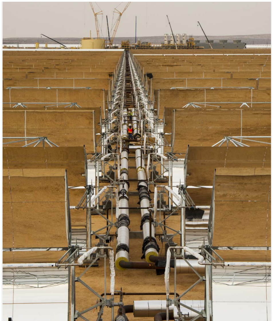
During construction, Mojave , created approximately 830 jobs. Photo Credit: Abengoa Solar, Inc.
