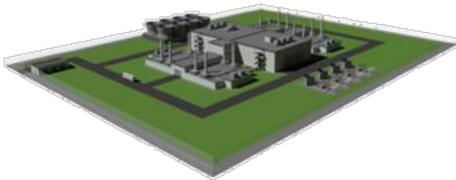
FIG. 1. Conceptual layout of a 4x55 MW(e) SEALER-UK plant
