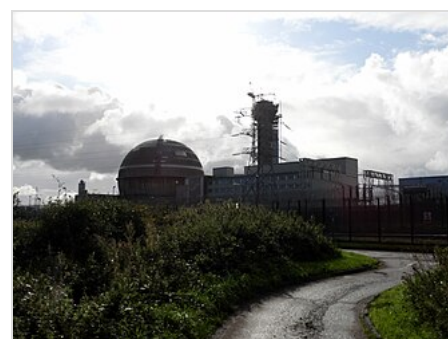
Pile 1 being dismantled in 2018
