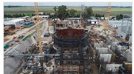
Status of the construction of the CAREM plant in July 2019
