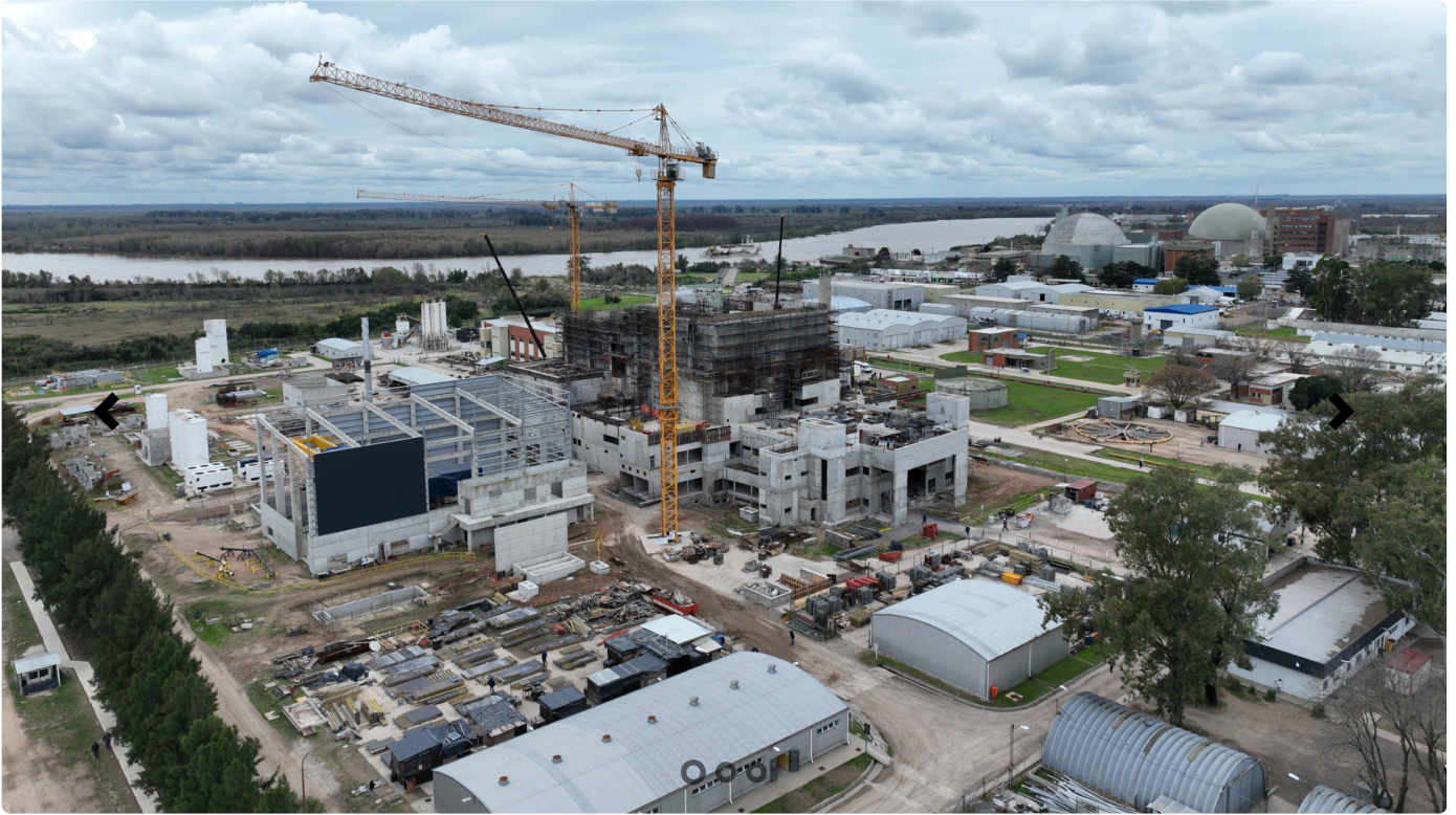
AUGUST, 2024. Advance status of the construction
