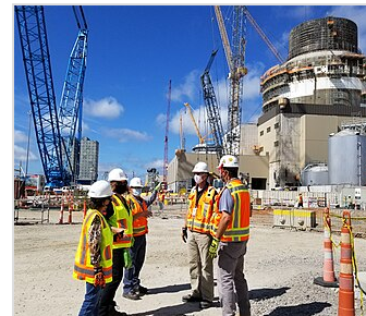
Vogtle Unit 3 under construction in October 2020
