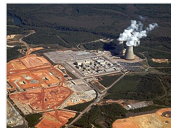
Construction underway at Vogtle, October 2011
