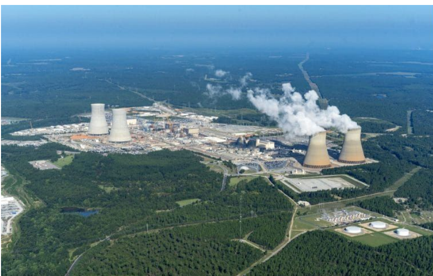
Vogtle reactor site in Georgia, with two operating units to the right and two AP1000 units under construction to the left; Tim Mousseau ©2019. Used with permission.
