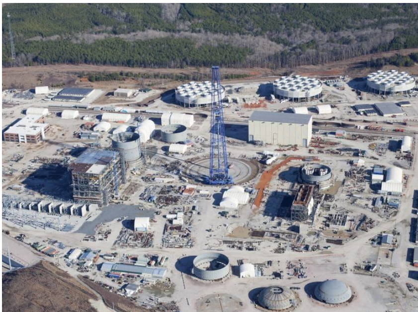
VC Summer abandoned AP1000 reactor site, with partially constructed turbine buildings and reactor containment buildings; Tim Mousseau ©2018. Used with permission.
