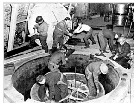
Allied soldiers dismantle the German experimental nuclear reactor at Haigerloch .
