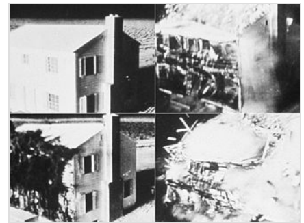
Frame house in 1953 nuclear test, 5 psi overpressure
