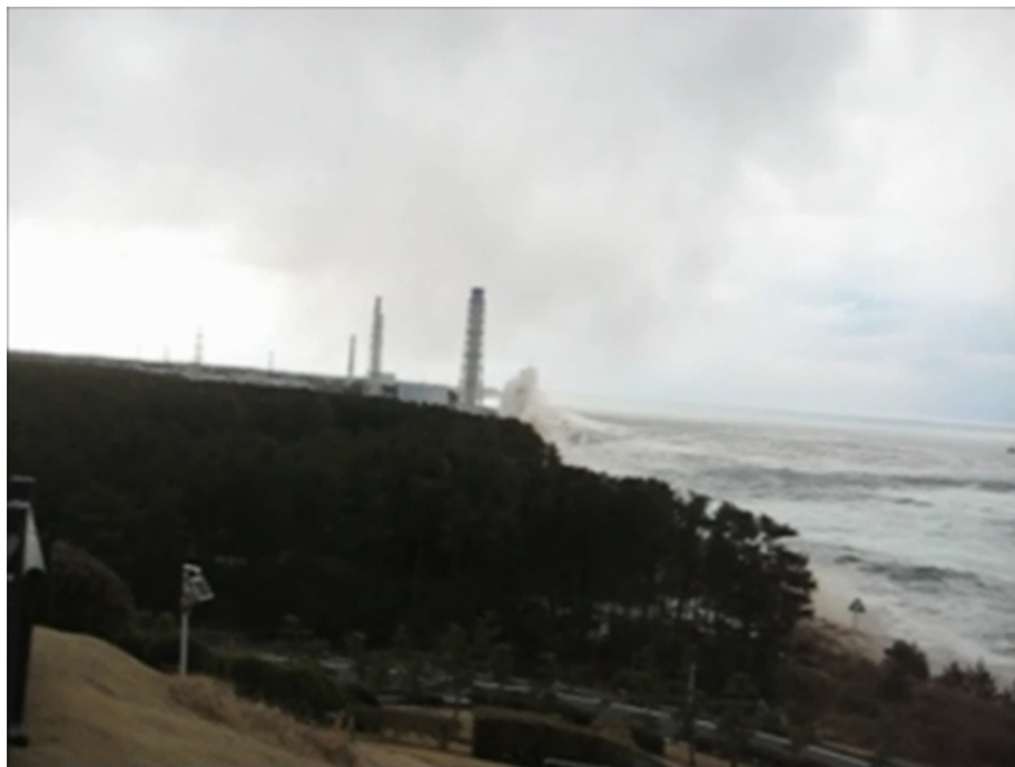
FIGURE 3.7 Photo taken looking north toward the Fukushima Daiichi plant on March 11, 2011. The photo shows the tsunami wave as it strikes the seaward side of the plant. Flooding can also be seen in the foreground of the photo. SOURCE: Courtesy of TEPCO ( http://photo.tepco.co.jp/library/110409/110409_1f_tsunami_1t.jpg ).
