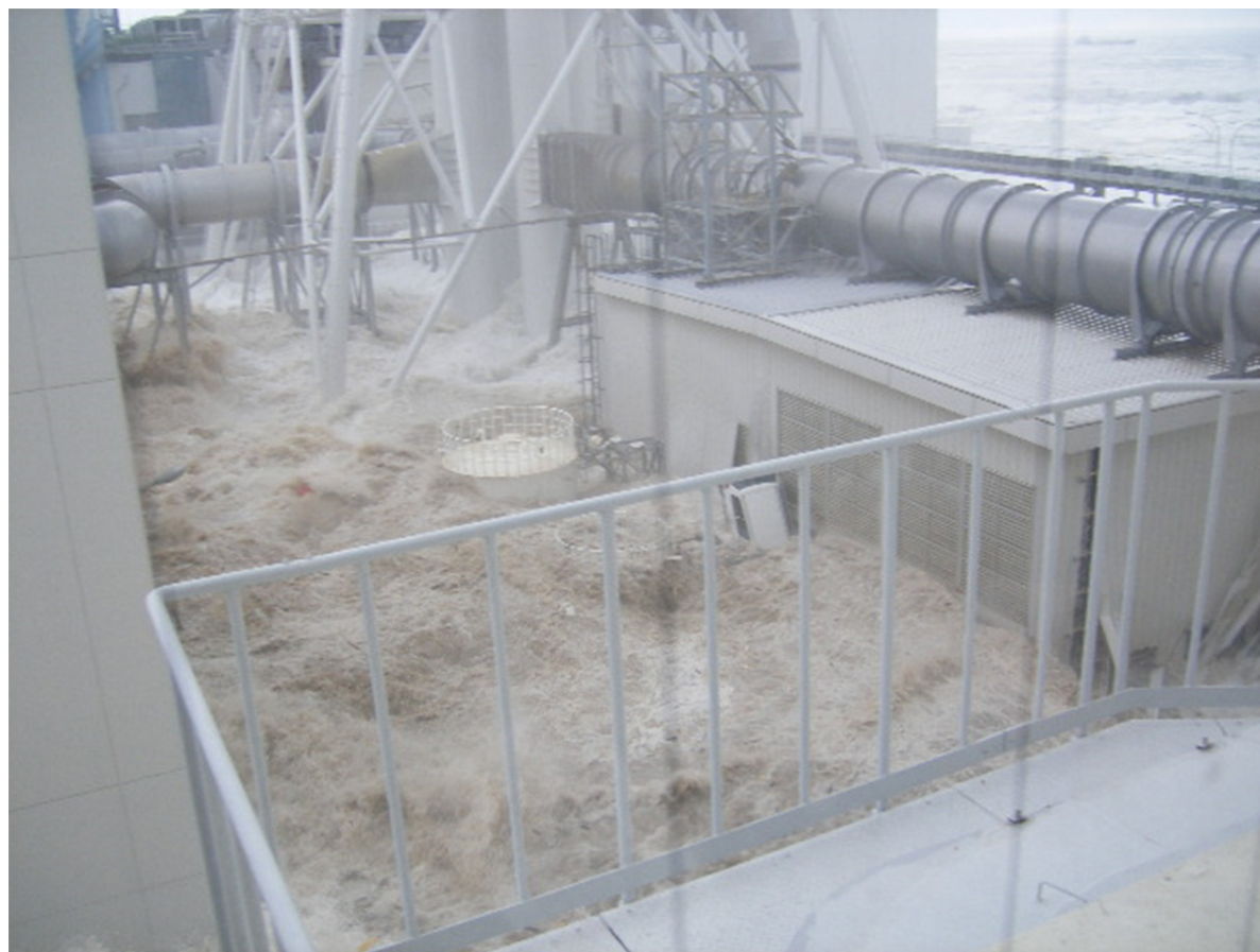
FIGURE 3.8 Photo showing flooding at the Fukushima Daiichi plant on the north side of Radiation Waste Treatment Facility on March 11, 2011. This facility is located south of Unit 4 (see Figure 1.2 in Chapter 1). Scale is indicated by the back end of a vehicle propped against the metal door. SOURCE: Courtesy of TEPCO ( http://photo.tepco.co.jp/library/110519_2/110519_1_4.jpg ).
