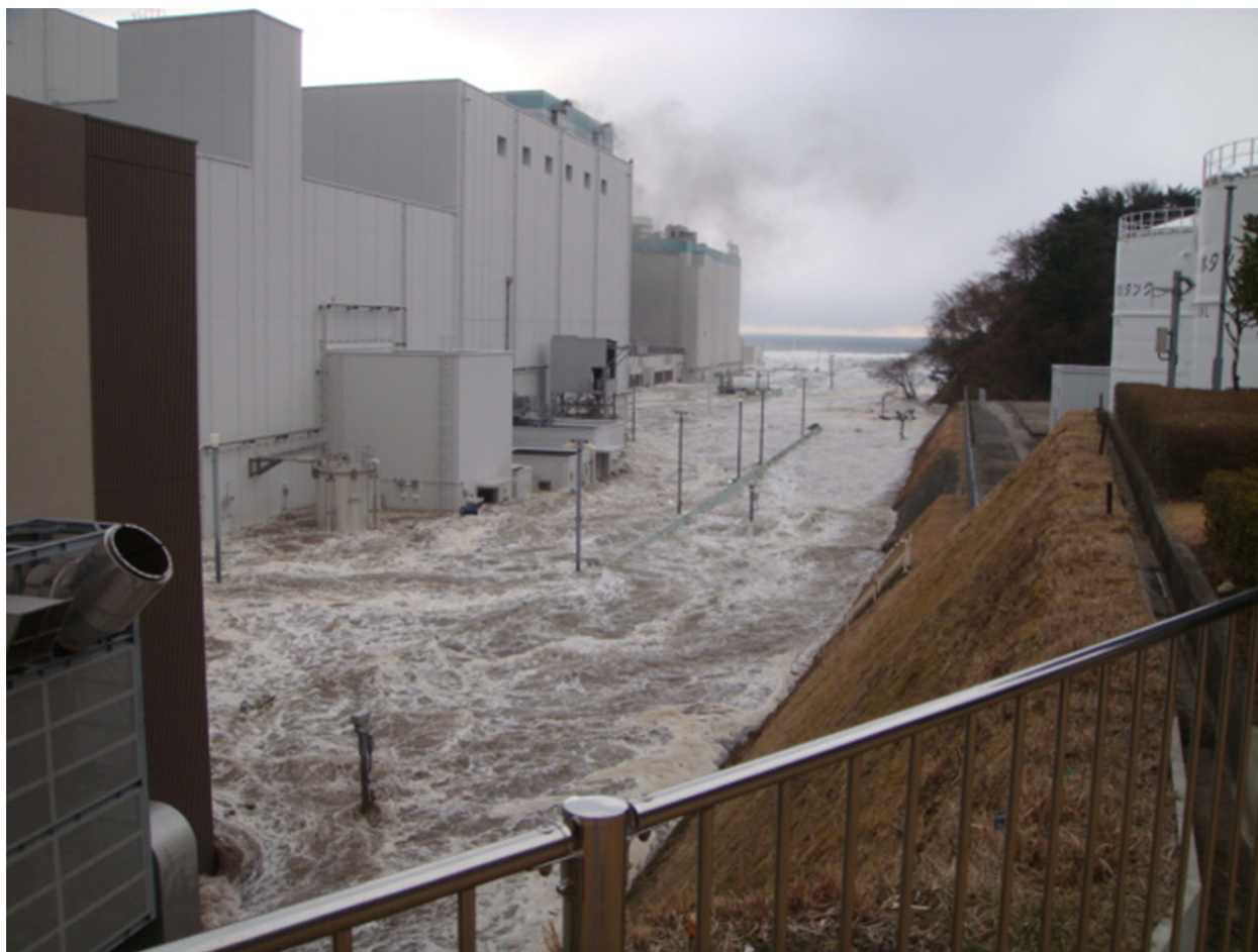
FIGURE 3.11 Photo showing flooding of the Fukushima Daini plant adjacent to Unit 1 during the March 11, 2011, tsunami. Flooding depth was between 2-3 m. SOURCE: Courtesy of TEPCO ( http://photo.tepco.co.jp/library/110411_3/110412_2f_tsunami_6.jpg ).
