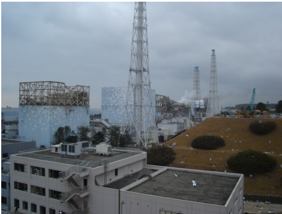
FIGURE 1.3 March 16, 2011, photo of the Fukushima Daiichi Nuclear Power Station showing damaged Units 1 (foreground), 3, and 4 reactor buildings. SOURCE: Courtesy of TEPCO ( http://photo.tepco.co.jp/library/110316/110316_1f_chijou_2.jpg ).
