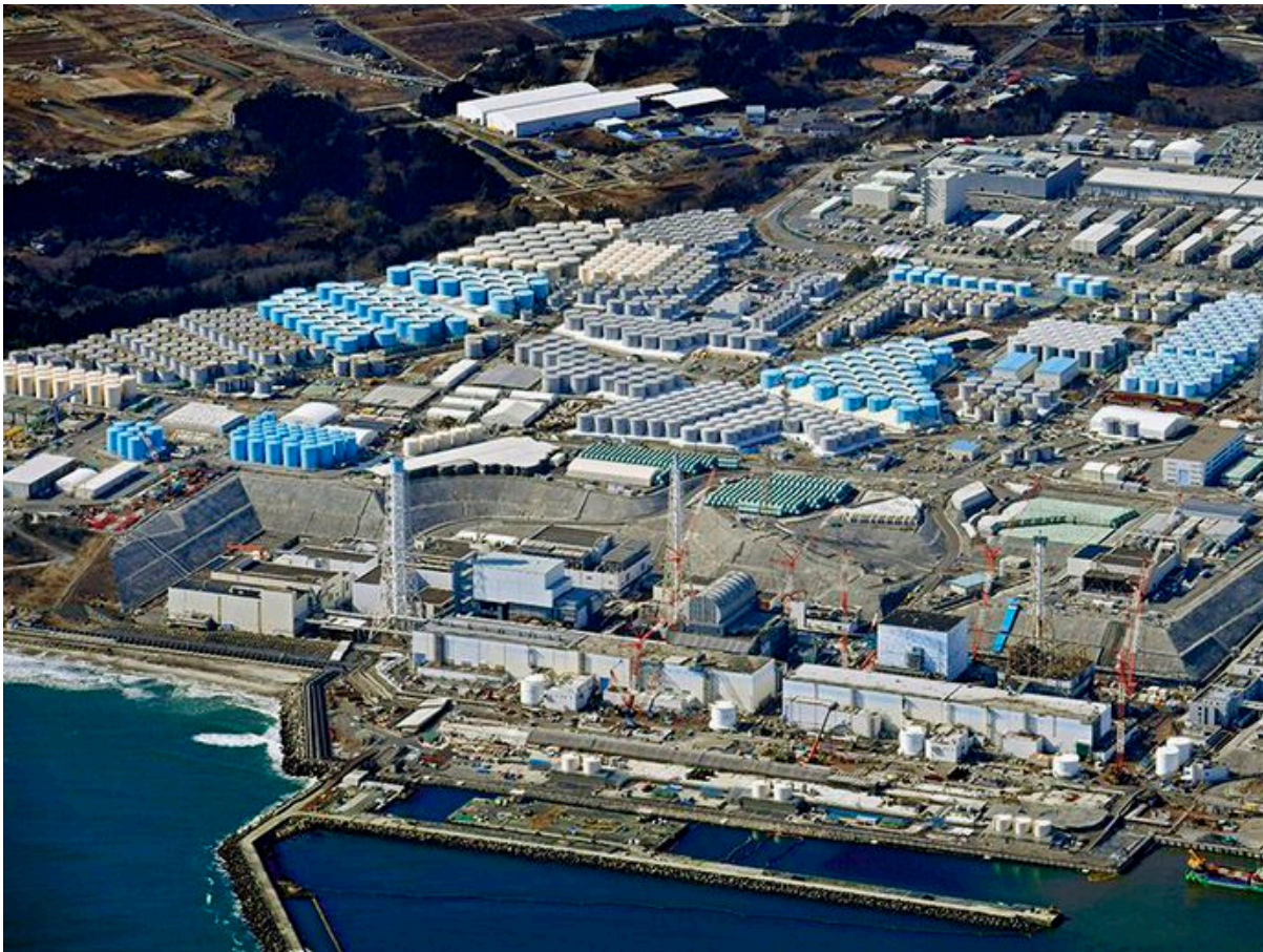
Current aerial view of the Fukushima Daiichi plant (2020)
