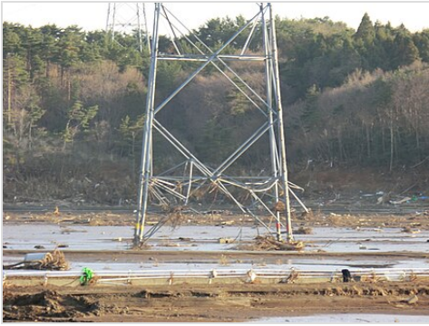
A damaged transmission tower and severed power lines in Minamisōma, Fukushima
