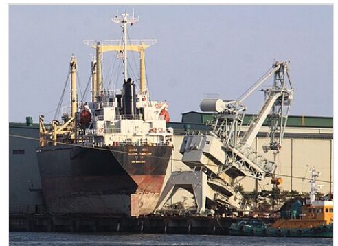
A damaged crane stands next to a ship lifted onto the docks at Sendai's port.
