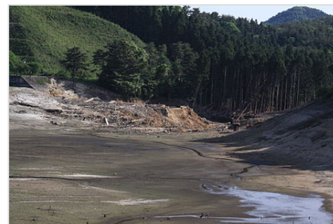
Dam failure at Fujinuma
