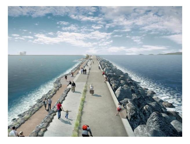
Lagoon power works by using a system similar to a lock to get different water levels either side of the huge wall. The doors are closed to allow water to come into the lagoon as the tide rises, and then when it goes out again the doors are opened and the water pushes past turbines and generates electricity.
