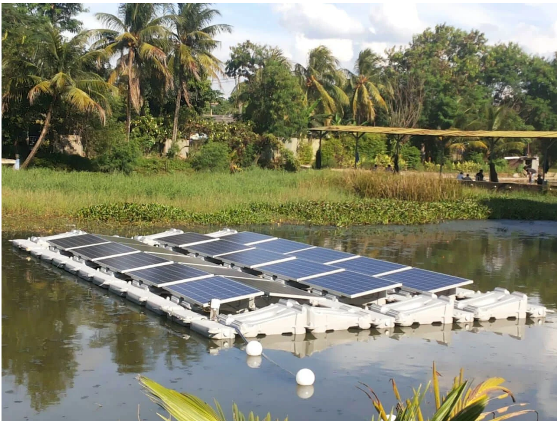
A solar pilot project on a flood control waste pond in Indonesia. Credit: Ciel & Terre International
