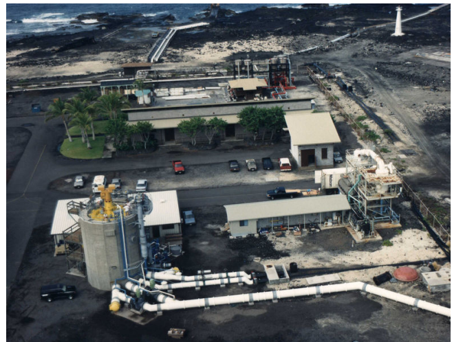
An experimental OTEC plant on the Kona Coast in Hawaii
