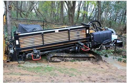
Geothermal drill machine in Wisconsin, USA
