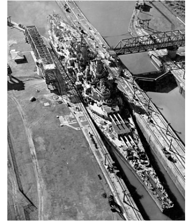
USS Missouri , one of the Iowa -class battleships, makes a very tight fit as she passes through the Miraflores Locks of the Panama Canal in October 1945.
