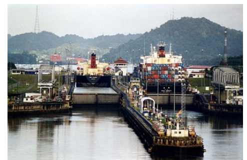
Two Panamax ships seen almost touching the walls of the Miraflores Locks.
