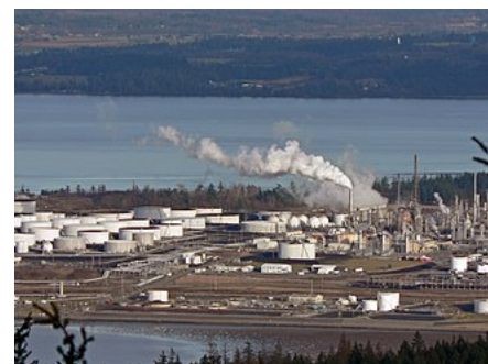
Storage tanks and towers at Shell Puget Sound Refinery (Shell Oil Company), Anacortes, Washington
