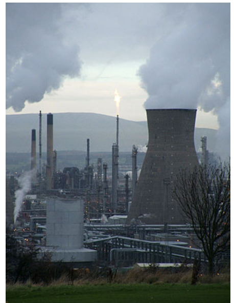
Grangemouth Refinery , in Scotland
