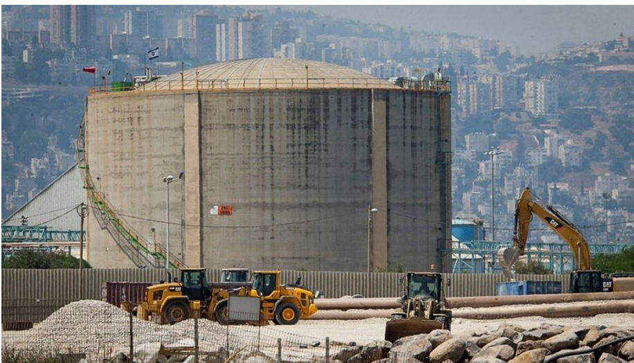
Figure 14: Ammonia tank at Haifa. Source: The Times of Israel 61
