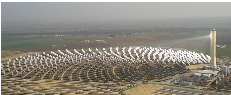
Mirrors powering the PS10 solar boiler in Spain [31] .
