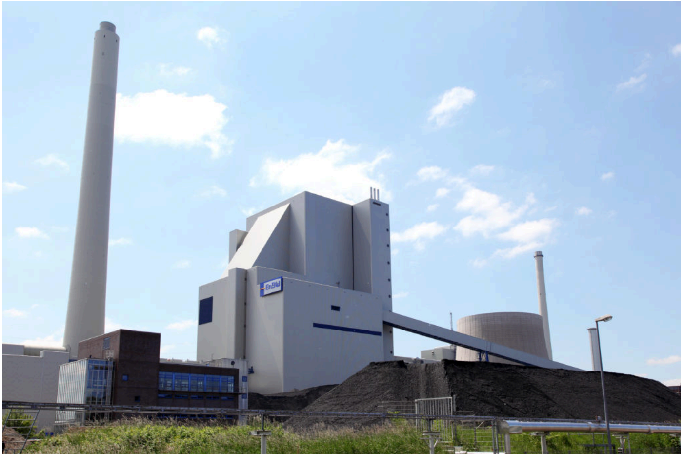
An exterior view of the RDK 8 power plant. Image credit: GE Power
